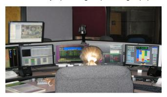
A typical Dispatch Console includes 8 computer screens, 2 computer keyboards, 3 computer mice, a multi-line phone system, 2 radio speakers, 2 digital playback recorders, 2 headset jacks and a foot pedal to transmit on the radio. The consoles raise and lower to accommodate a sitting or standing work preference.
